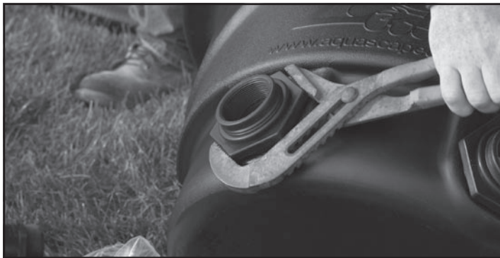
Fig. 1 Attach bulkhead fitting.
