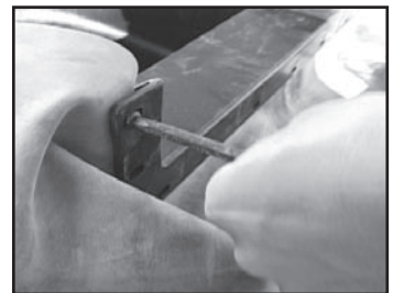
Fig. 10 Begin threading one of the screws into the filter.
