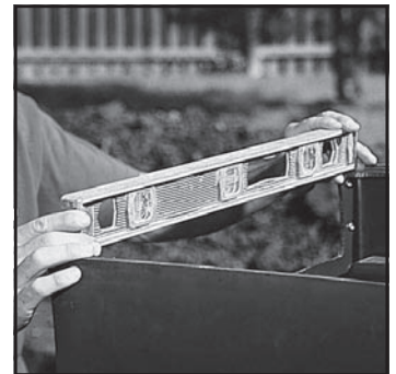
Fig. 3 Level the BIOFALLS® filter side to side as well as front to back.
