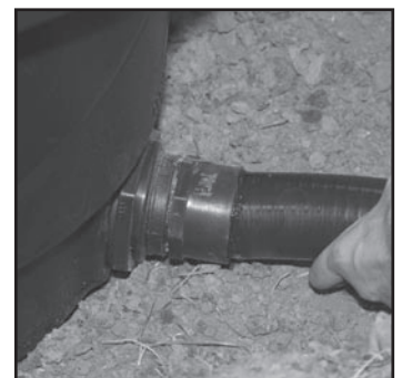
Fig. 4 Finished bulkhead assembly.
